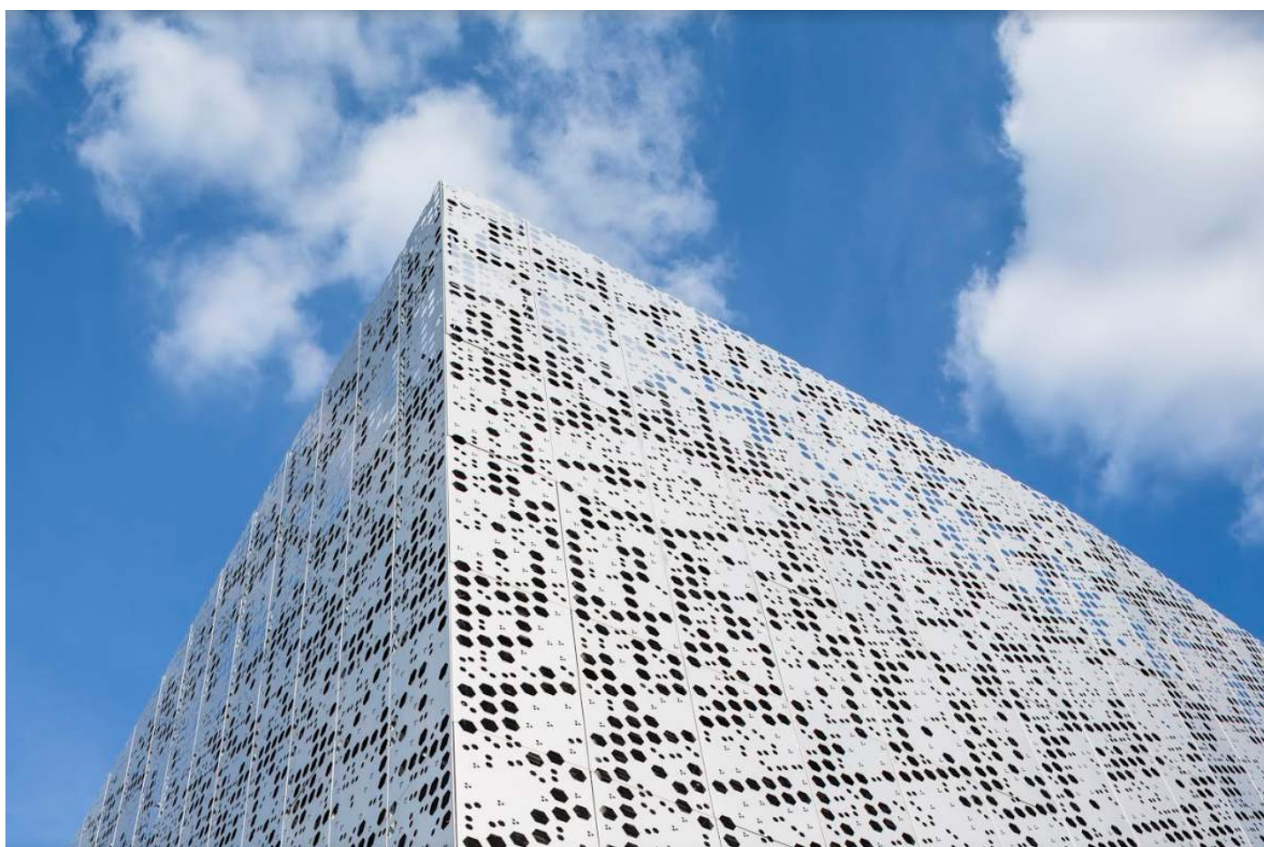
Conservation center for the departmental archives of the Nord, Lille, France; de Alzua+ /ZigZag Architecture © Sergio Grazia Stainless steel used: Aperam 304 with Uginox Mat surface finish
