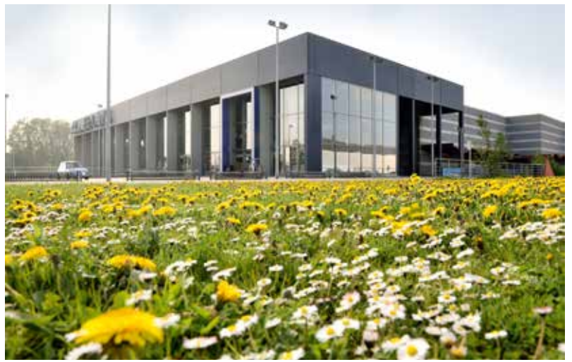
Energy-saving steps are taken when renovating existing complexes.
