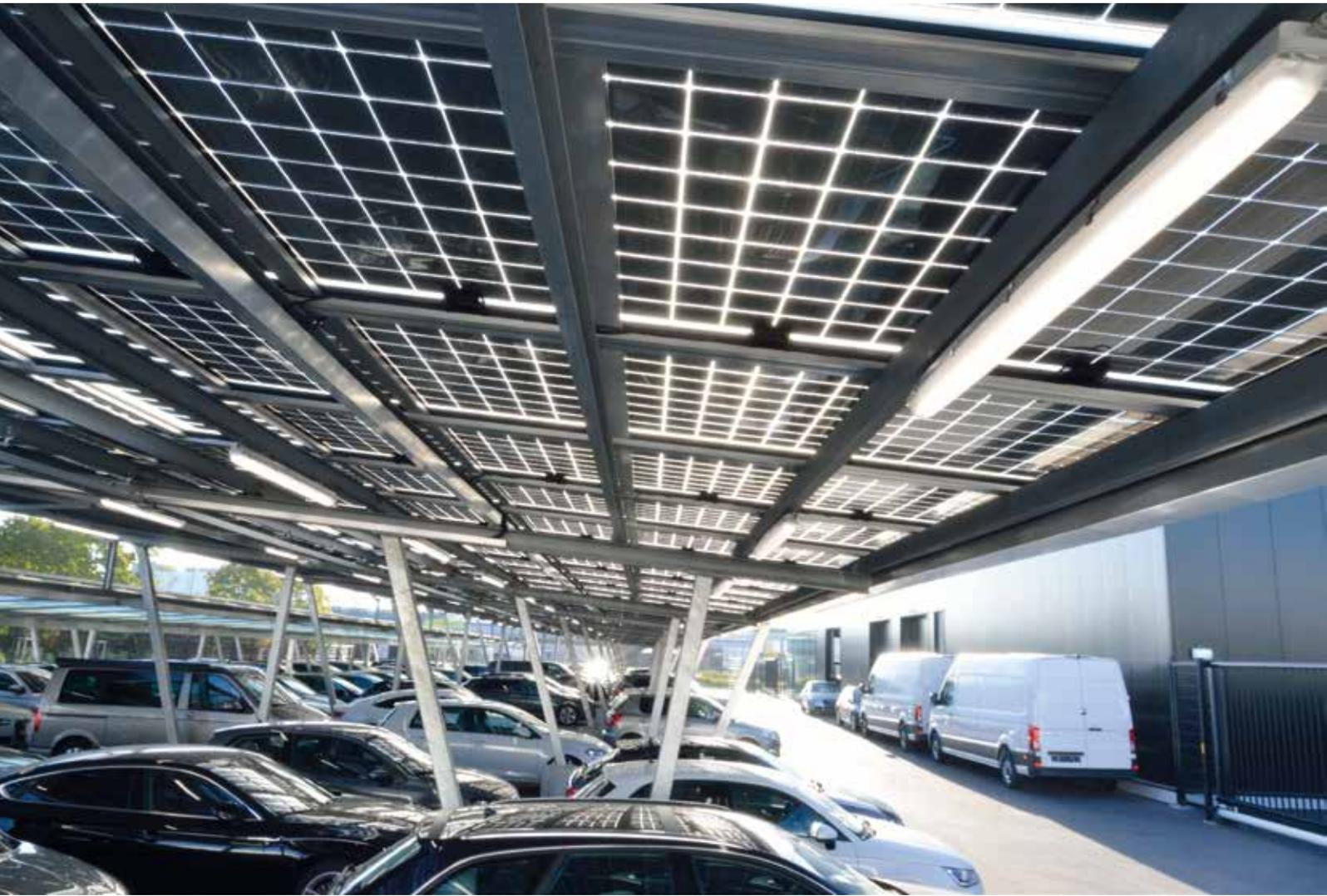
*Photovoltaic carports have been installed in the new Wondercar bodywork building in Drogenbos. The produced electricity reaches 301 MWh per year, allowing to recharge between 50 and 100 VW e-Golf or almost 150 Audi Q7 e-tron a day.*
