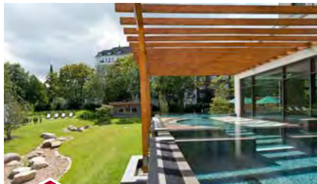
Sport and well-being centre - Uhlenhorst (DE)
