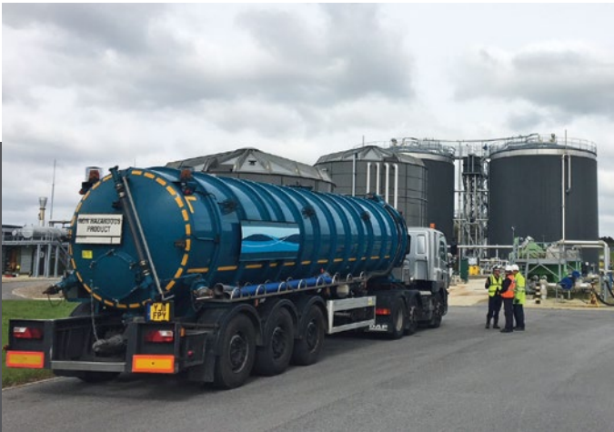
Tanker arriving at our sludge treatment centre at Worksop, north Nottinghamshire.
