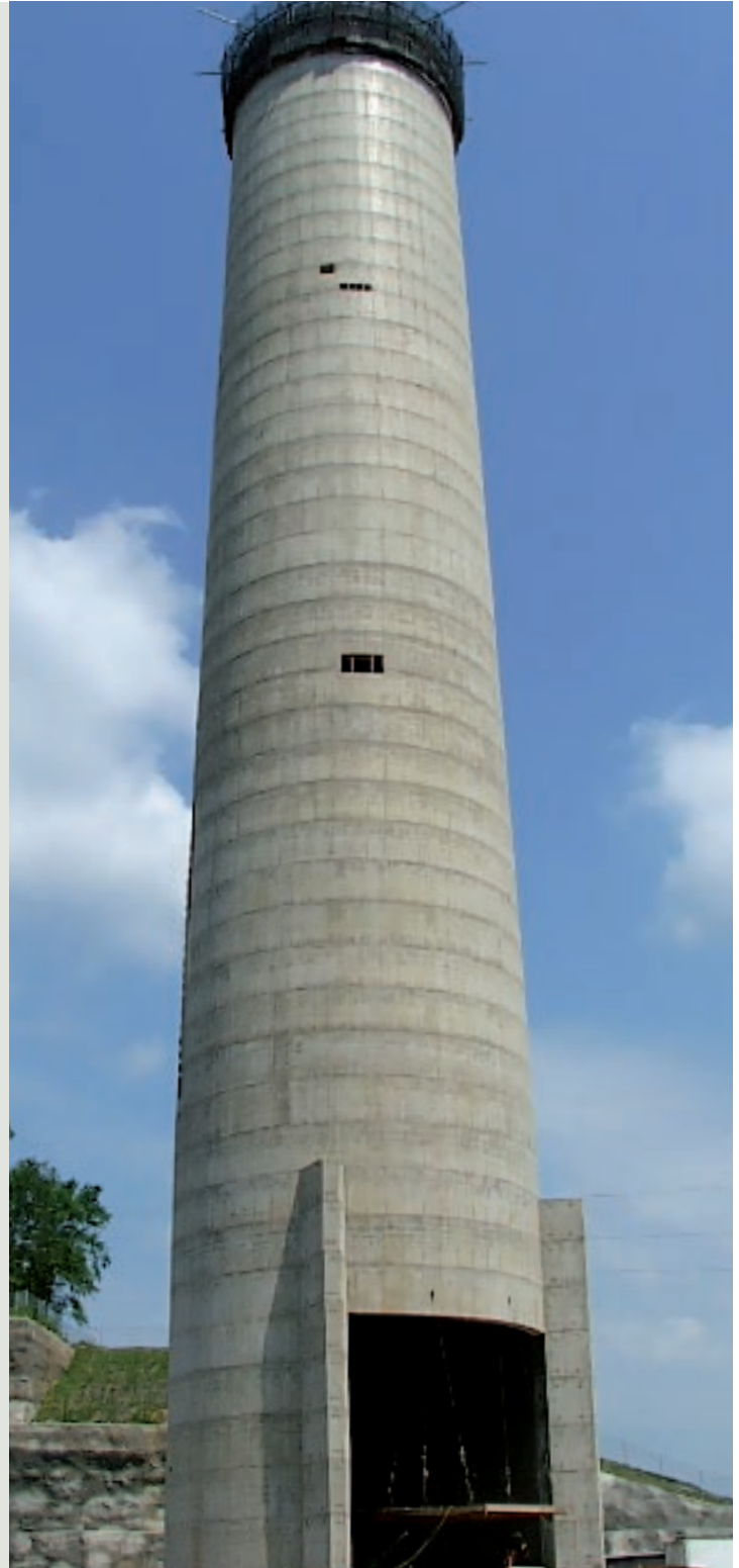
Construction of a concrete chimney in USA
