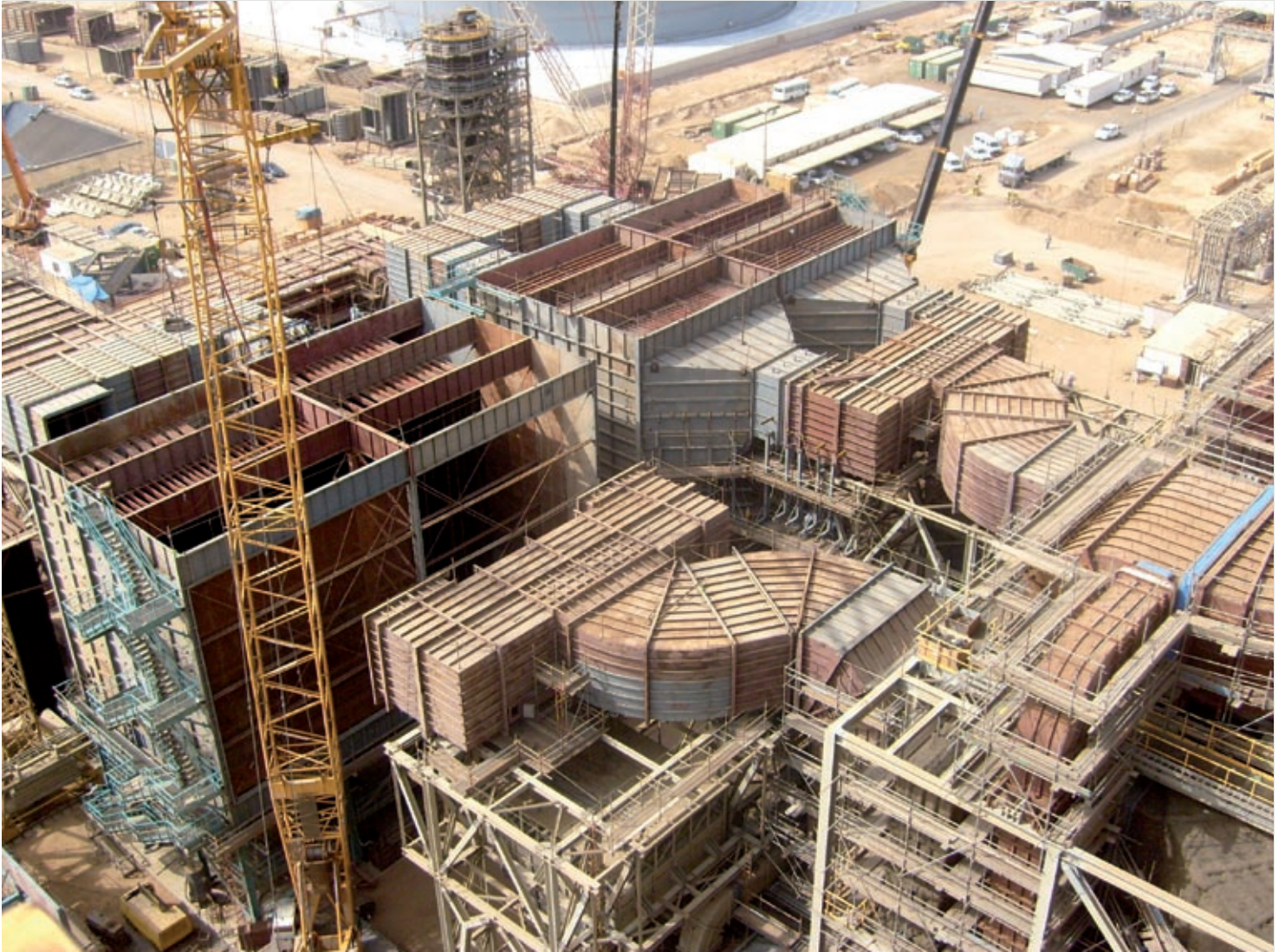
Construction of an ESP in a petrochemical plant in Saudi Arabia
