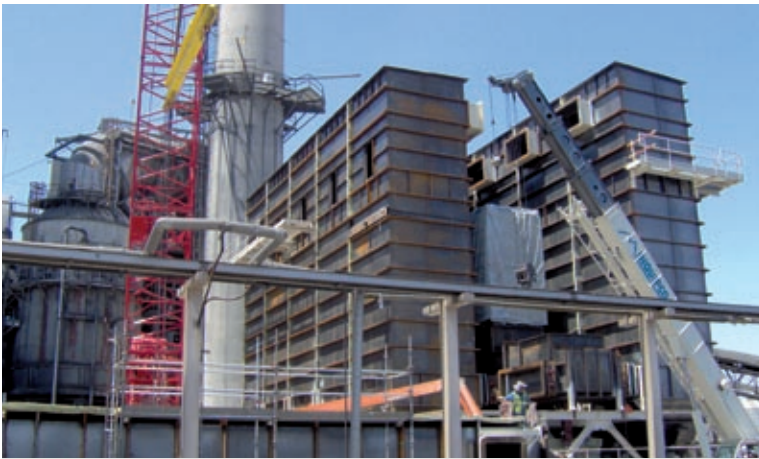
Fabric filter under construction in a power plant in USA
