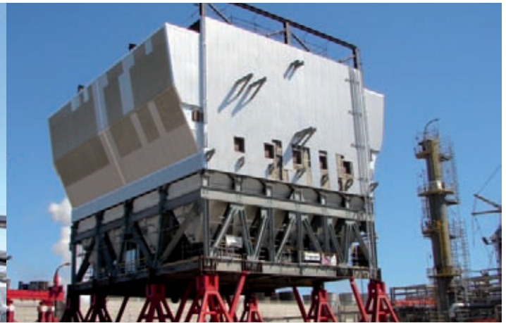
A new ESP is put in place in a refinery in USA
