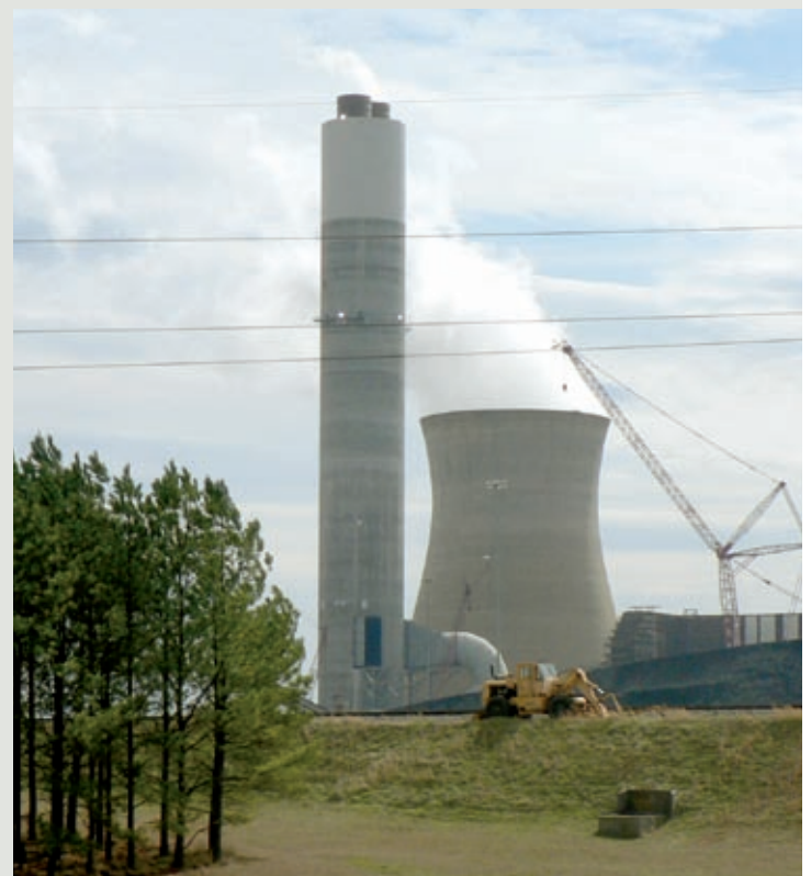
Chimney in a power plant in USA
