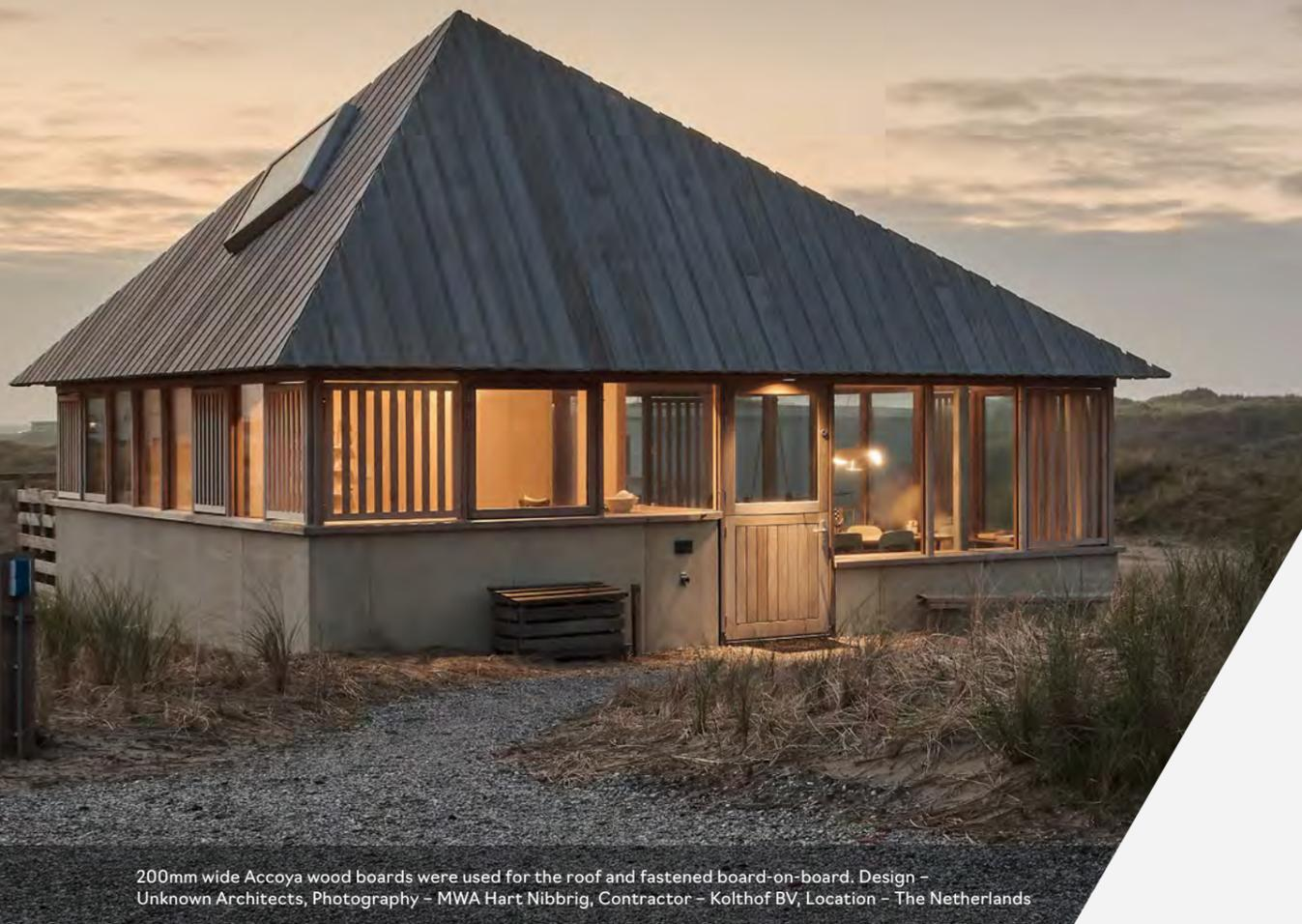
200mm wide Accoya wood boards were used for the roof and fastened board-on-board. Design – Unknown Architects, Photography – MWA Hart Nibbrig, Contractor – Kolthof BV, Location – The Netherlands
