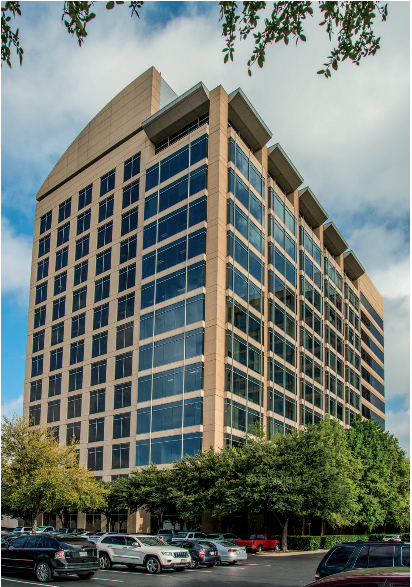
Dallas, Galleria North Tower II
