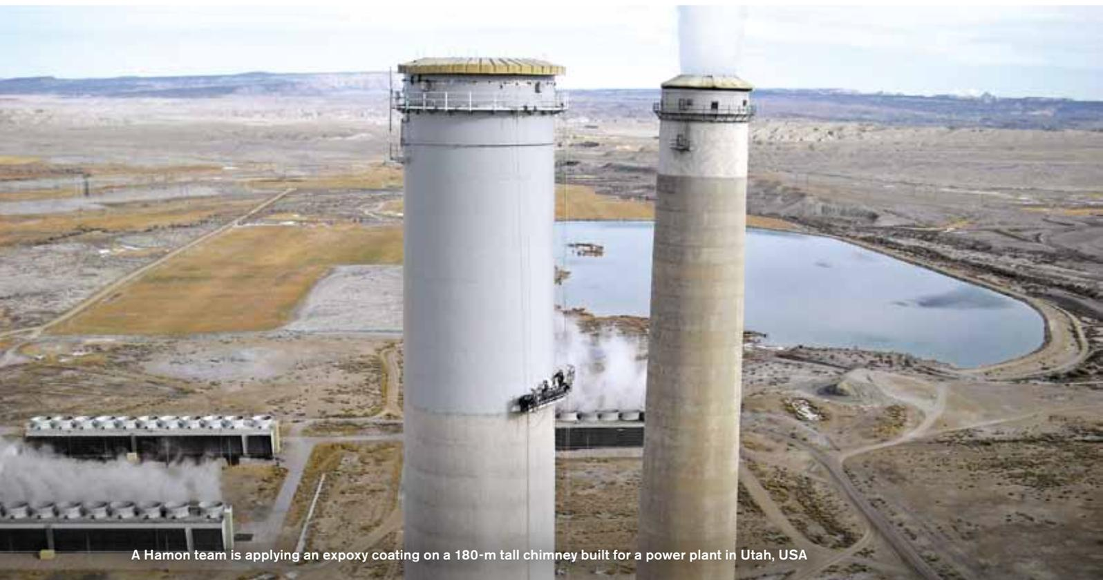
A Hamon team is applying an epoxy coating on a 180-m tall chimney built for a power plant in Utah, USA
