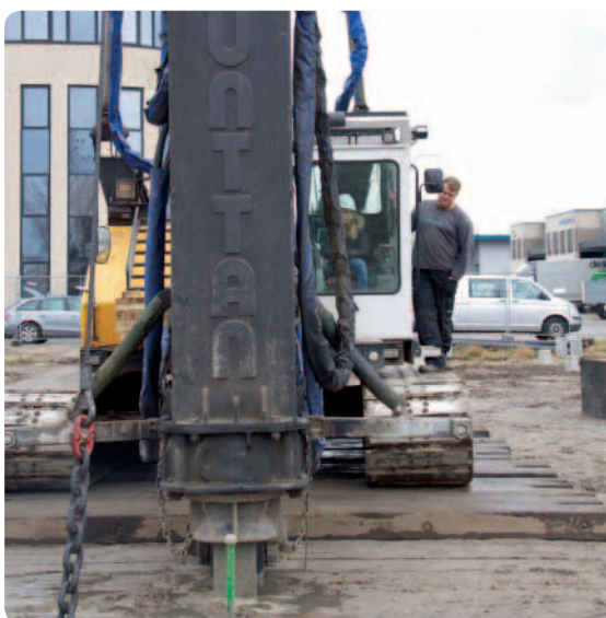
30 March 2010: Laying the foundation of the new Fagron building
