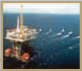
First tension leg platform (TLP) Hutton, UK North Sea (1984)
