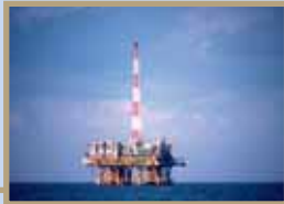
First fixed platform Cognac, Gulf of Mexico (1977)
