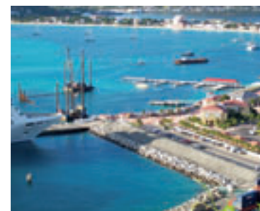
The port on the island of St. Maarten in the Netherlands Antilles is being made suitable for large cruisers. In the future, six ships a day will be able to dock at the new pier. The progress of the work can be tracked on www.bnpa.eu .
